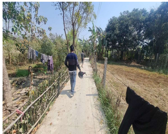
After Construction, Surya Path East Galli road towards Manoj Guptas House.
