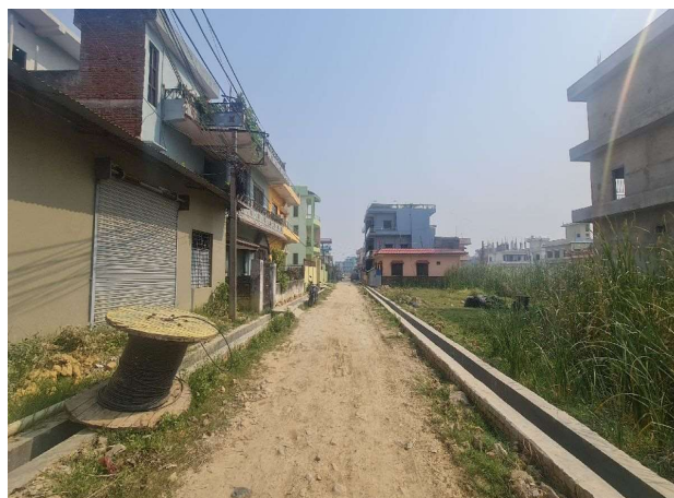
After Construction, Dipjyoti Path
