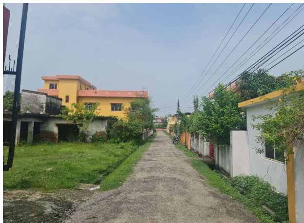
Before Construction, Lekhnath Path
