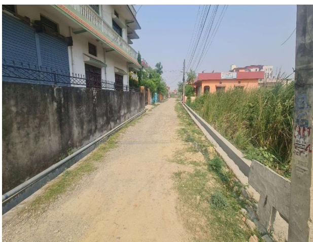
After Construction, Friends Colony
