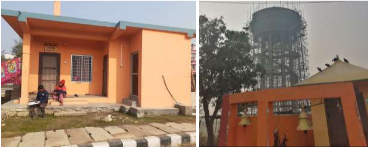
Figure 3-14 water supply, Well no -5 in ward no- 3 and Over Head water tank in ward no -4
